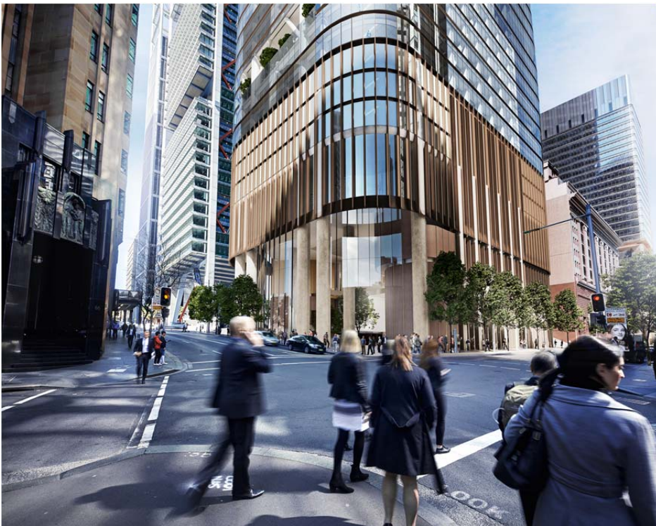
Figure 74 – View of proposed illustrative scheme from Richard Johnson Square looking south down Castlereagh Street
