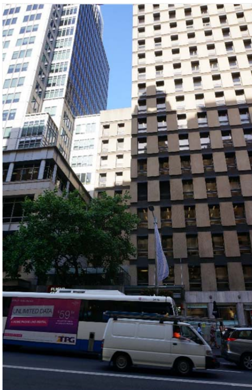
Figure 31 – the South Site building adjoining to 60 Castlereagh Street
