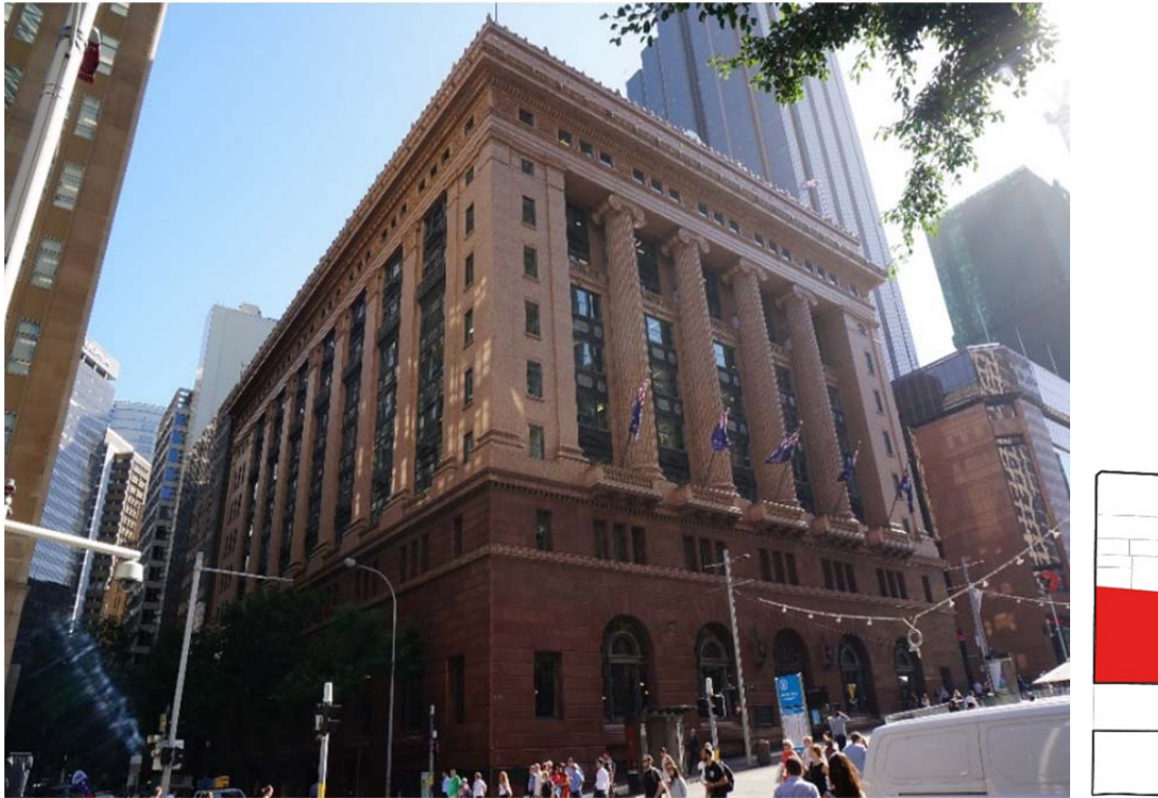
Figure 8 – 50 Martin Place as viewed from Martin Place and Castlereagh Street
