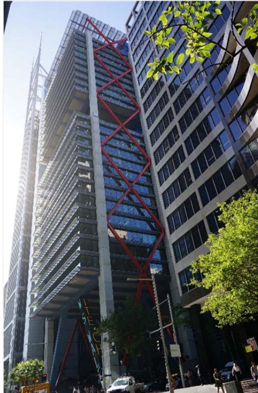
Figure 28 – 8-12 Chifley Square, as viewed from the corner of Hunter and Chifley Square
