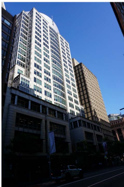
Figure 30 – 60 Castlereagh Street, as viewed from Elizabeth Street
